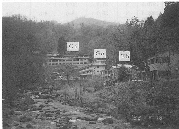
Photo-1 A general view of Motoyu Spa in 1992
