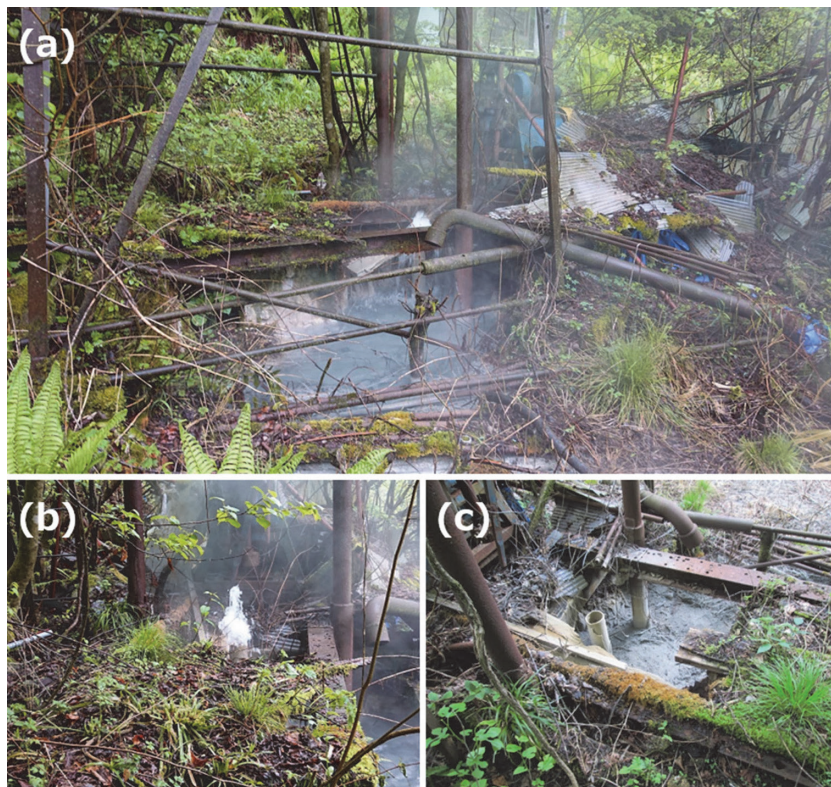
Fig. 3 Photograph of the abandoned well. During the abnormal discharge (May 19, 2020 ; a and b). After the discharge stops (May 27, 2020 ; c).
