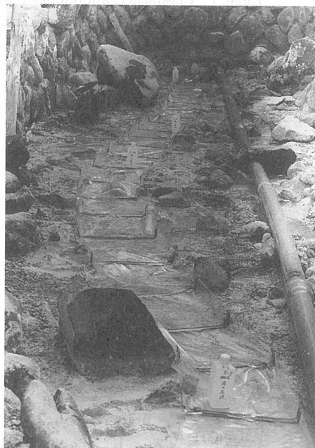
Fig. 2 Photograph of the artificial outflow set the U-type sheet onto the natural outflow of the Yunohanazawa hot spring.
